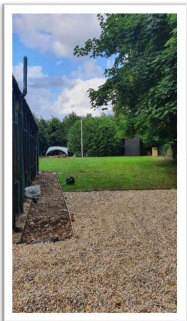
To the front of the HQ, we've finally completed the works associated with the drive and entrance, and we've managed to level the lovely hardcore and put the stones across the top for easier access. We also have a few concrete paths to construct to the right of the building and to the front of the building, which will run to the containers and to the fence. We will also in the future be constructing a new access gate between the containers.
